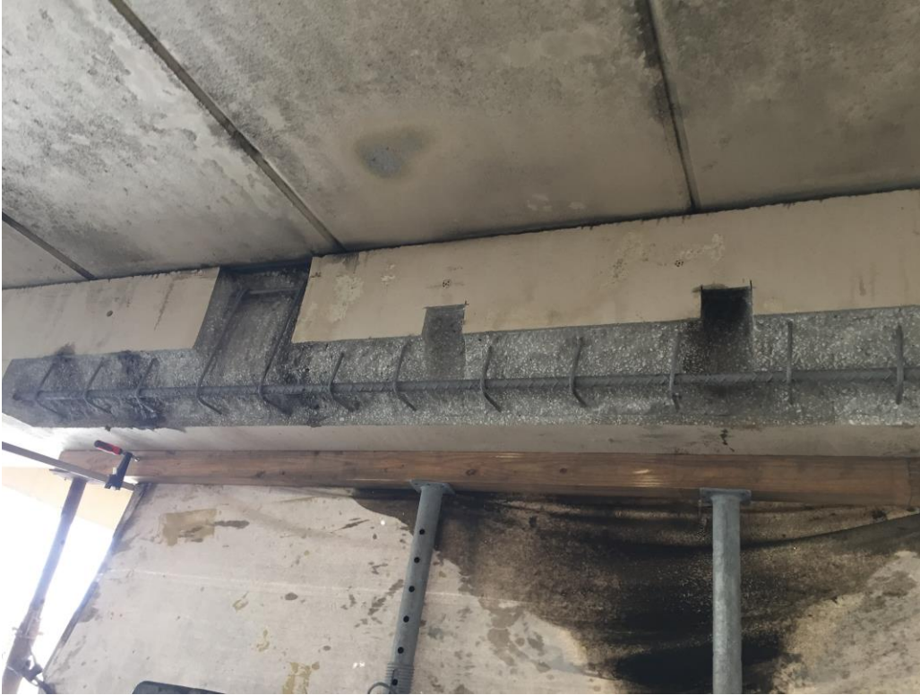
Picture 1: Excavation approved to be cast
