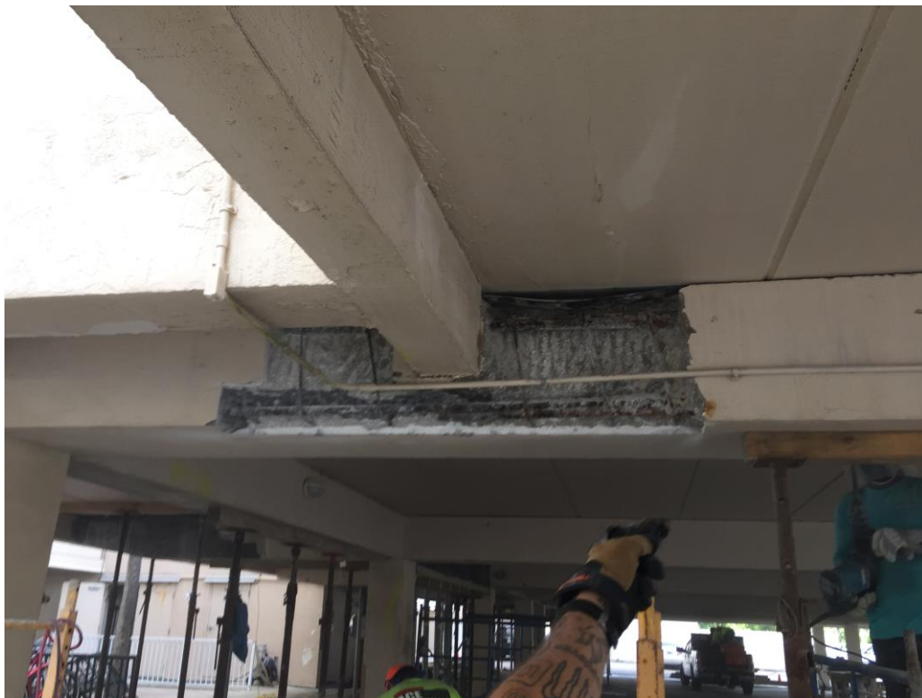
Picture 3: In-progress demo
